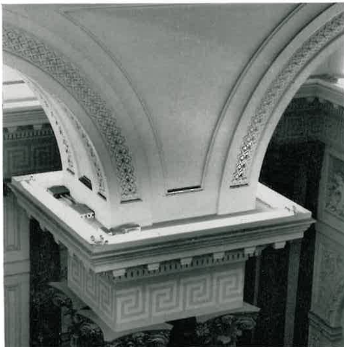
Fluorescent lamps are mounted on the existing cornices, a metal upstand screening them from view.
